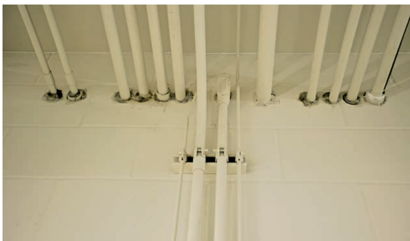
FIGURE 18. Caulking around Service Intrusions*
